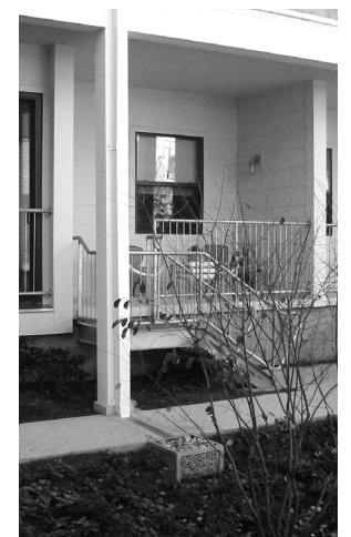
downspout detail, Elevation 314
