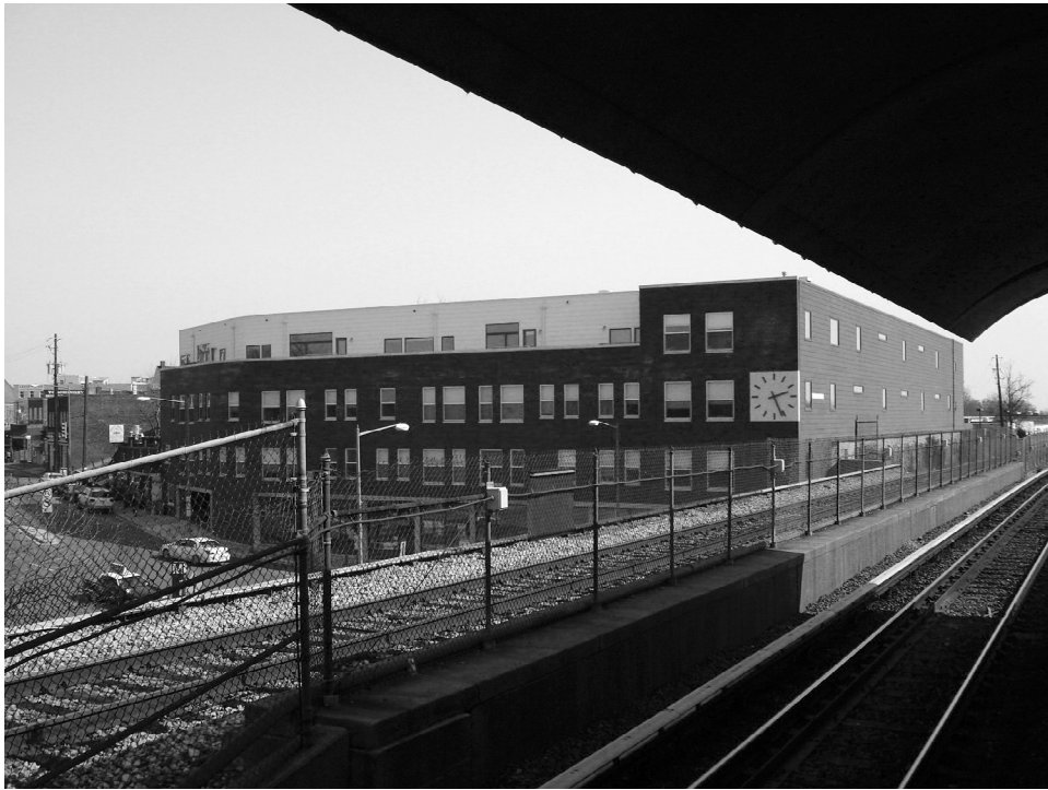
view from adjacent metro stop, Elevation 314
